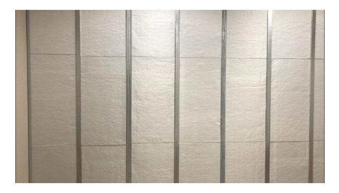
**Attention**: press lightly between the panel and the panel to eliminate any gaps. It is possible to seal the joints by taping them with the silver "American" type ISOL-TAPE adhesive tape.
