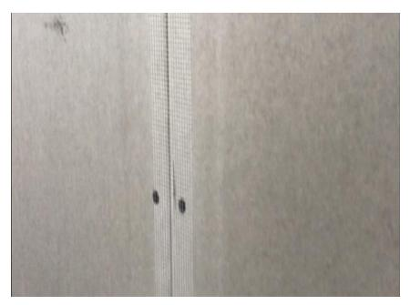
After drying, check that there are no imperfections or micro irregularities along the joint; for this grouted purpose, drag the spatula across the joint, placed transversely to the axis, and remove any roughness with the same spatula or a special fine-grained pad with sandpaper.
