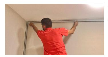
Apply the upper guide to the ceiling, with suitable fixings for the support, placed at a maximum distance of 50 cm.
