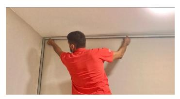
1st step: installation of the "U" guide and fixing the riders
