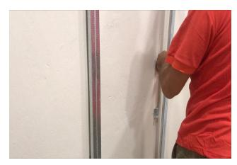
Note: if ducts are to be passed, use appropriate uprights of the necessary thickness to pass any systems. If the wall is high and it is necessary to join the profiles, make an overlap.
